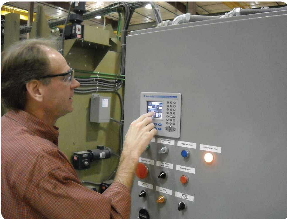
Panel with Optional PLC Controls
